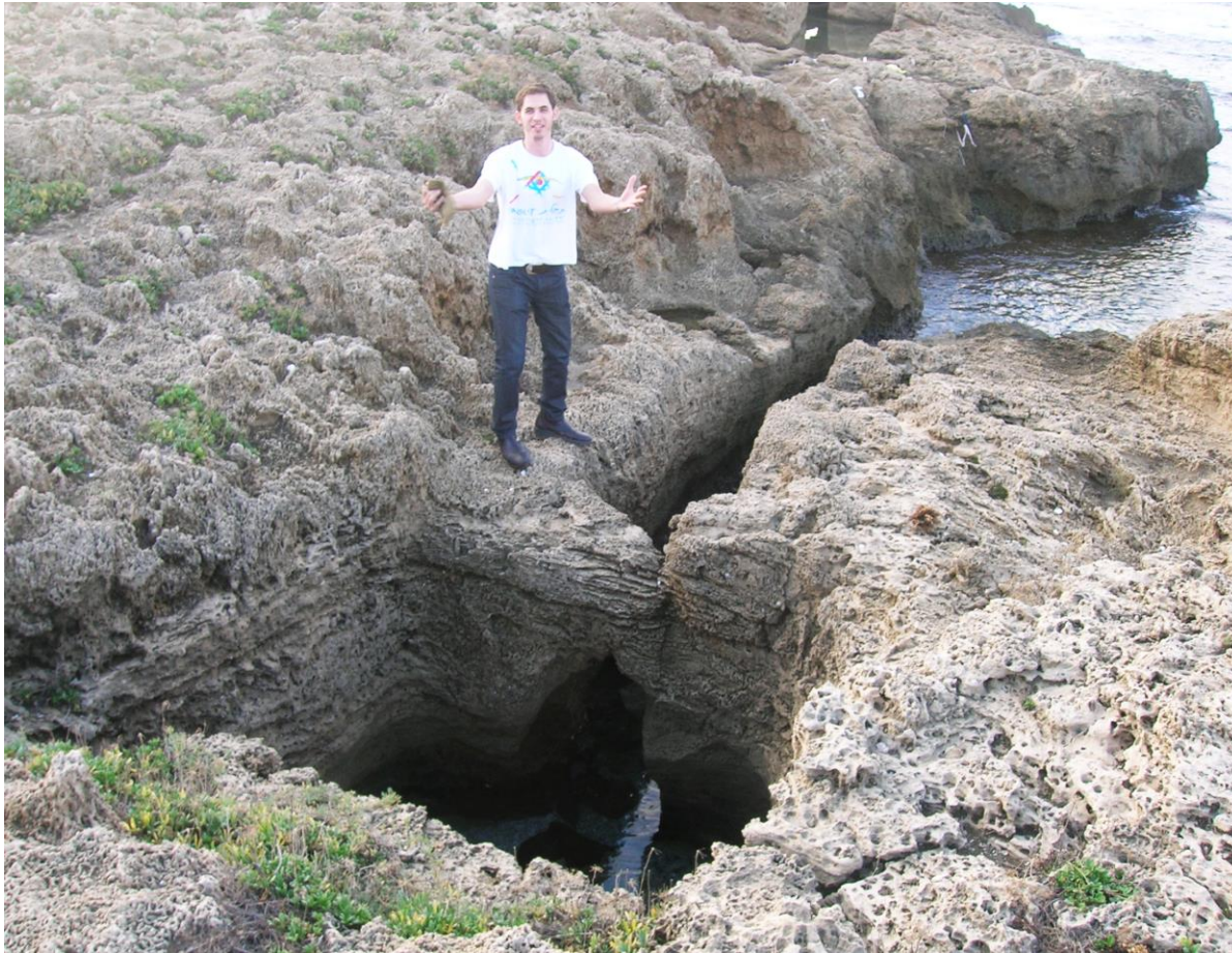
Sea-water well (pumping station) of Installation for salt production, Carmel coast
